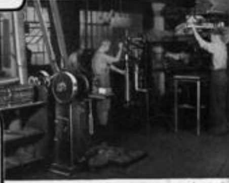
A partial view of the Chime and resonator tube stock. In center is workman performing one of operations in tuning resonators.
