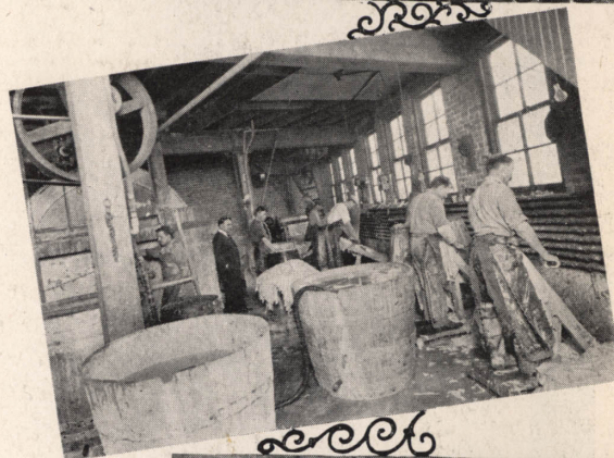
"Beam" House Work
