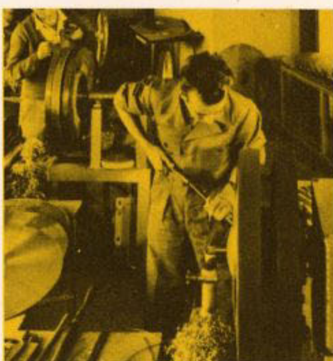
Precision, final machine spinning for beautiful finish.
