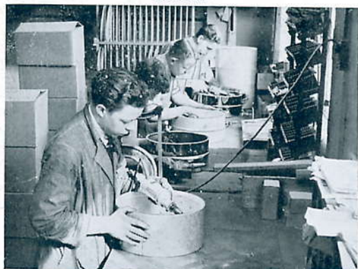
High-speed electric drills being used to prepare the shells for the tension rods and snare fittings.
